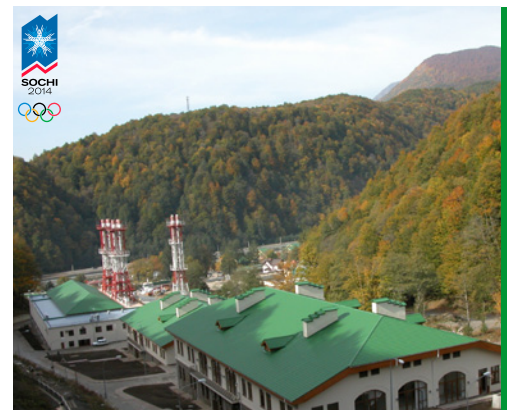
Six OP16 turbines installed at the 2014 Olympic Winter Games site in Russia
